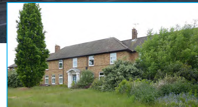
Existing disused building
