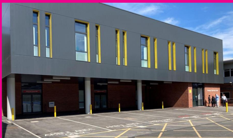
York Hospital's new A&E Department
