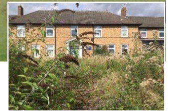
Bootham (top photo) Oakhaven (below)
